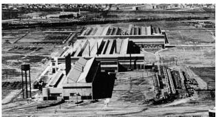
Figure 100: Section of the River Rouge Plant with sawtooth roof (Image Detroit Publishing Co. in public domain)
